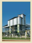
Client: Barralcool Location: Barra do Bugres, MT Process: Ethylic (integration with ethanol) Capacity: 50 000 T/Year Raw Material: Vegetable Oil
